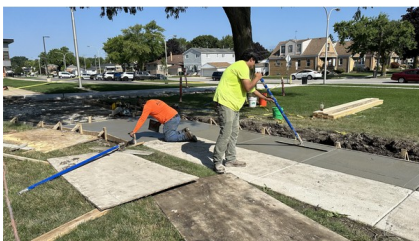
Sidewalk resurfacing in Elmwood Park District 401
