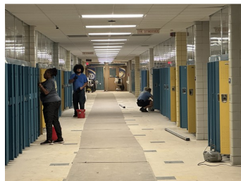
Hallway renovation in Lyons Township HS District 204
